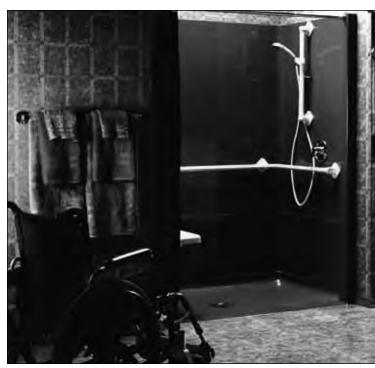
The slope of the floor in a roll-in shower is especially important so that water can be properly channeled into the drain. The area inside the shower needs to be carefully designed to allow room for maneuvering a wheelchair or wheeled shower chair. The ADA guidelines for roll-in showers call for a minimum of 30 inches in width and 60 inches in length.
