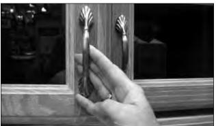
will maximize accessibility to wheelchair users. D-shaped hardware instead of knobs makes opening easier.
