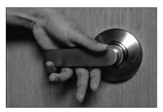
Keep in mind that lever-style door handles are easier to use than round knobs for someone with limited strength or dexterity.
